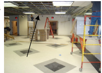
Early Friday: ceiling tile installation
