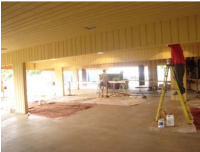
Final repairs being completed
